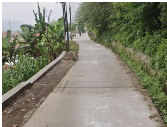
Figure 2: Existing Condition After Construction Source: Processed by Researchers, 2025
