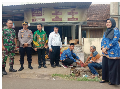
Figure 2. Tuban Regency Government and National Land Agency Conduct Earthquake Rehabilitation in Jenu District
