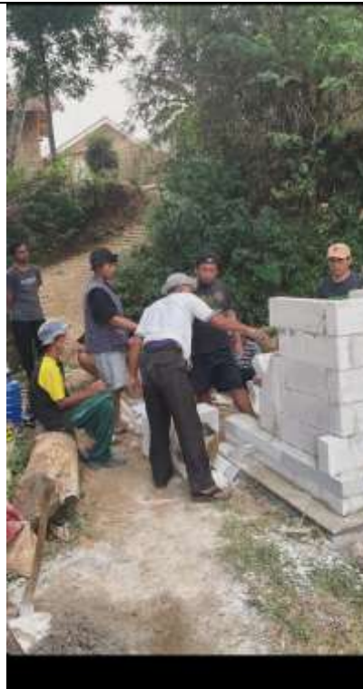
Figure 2. Participation of residents and students in the construction process of the Rocket Stove unit.
