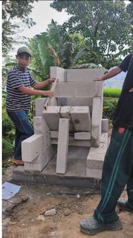
Figure 1. The frame assembly process and leveling measurement of the Rocket Stove structure.
