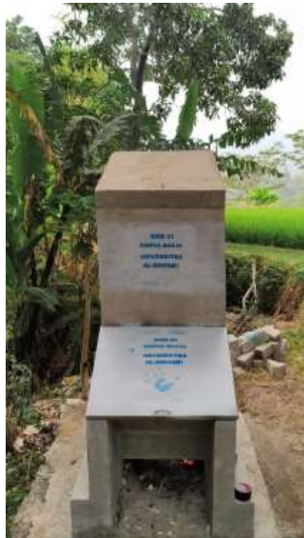
Figure 3. The completed Rocket Stove unit constructed on the RW 07 waqf land.
